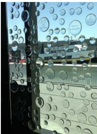
Bubble glazed unit with toughened glass A more expensive option, but lovely!
